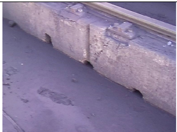
current drainage holes
