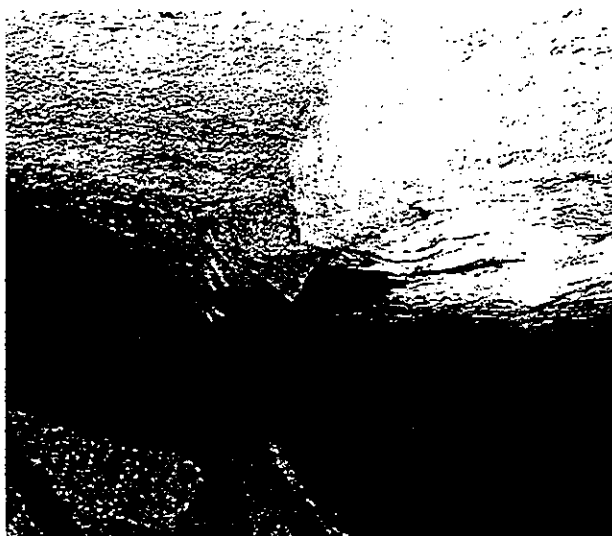
Feather-edging in a conglomerate roof, prevented from running into bord by roofbolts.
