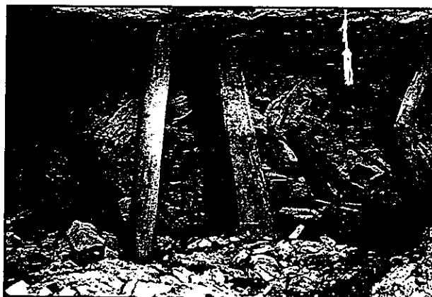
Well developed crush zone at the edge of a highly stressed coal pillar
