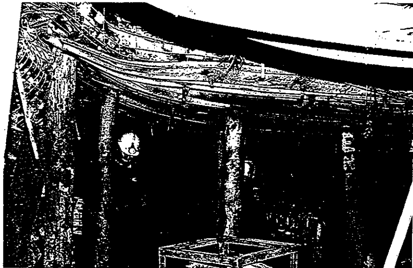
Weak roof which has given warning of impending failure, resulting in the progressive installation of mesh, bolts, straps, cross supports, legs, cablebolts and PUR.
