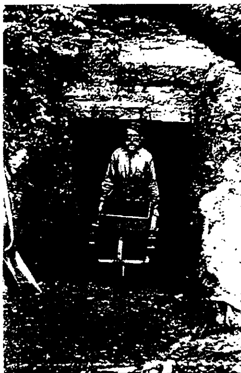
Wiley Mine Portal, 1898, illustrating the benefits of restricting bord width to control roof stability (reproduced from AusIMM Monograph 21 with permission from photo source, Mr. Jack Southern).
