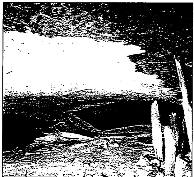
A feather edge in massive sandstone roof which has run down the bord for almost 15m. Note the low angle stress induced curved fracture plane tapering to a razor edge.
