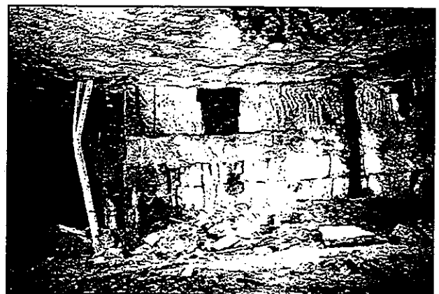
Vertical splitting induced in a coal pillar as a result of a soft band being squeezed out of the middle of the pillar
