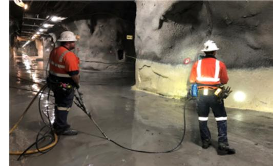
**DSI Silcrete** – potentially a system to improve the way we support ribs and remove support for extraction
