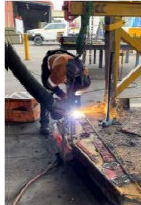
Fume extraction hood
