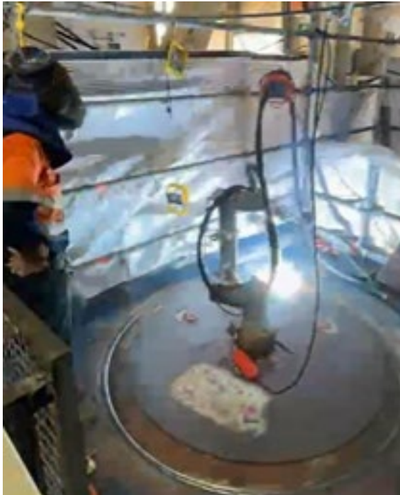
Robot performing weld repairs
